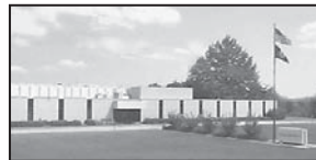
300 Industrial Park Road Farmville, VA 147,000 ± SF Manufacturing Sale - $2,100,000 Jason Hetherington, Bruce Milam
