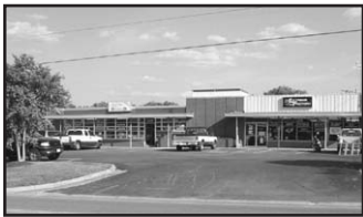
8007 Mechanicsville Tpk 9,669 SF Lease - $10.50 MGRS Bill Mattox
