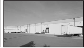
Airport Center I 5200 Anthony Road 95,545 SF Sublease - $3.95 NNN Jason Hetherington, David Williams
