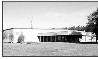
NEW Multi-Function Industrial Facility 13167 Telcourt Road 124,350 SF For Sale David Williams
