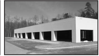
NEW Phoenix Business Center 713 W. Hundred Road 2,200 to 16,000 SF $10.00 + Utilities Greg Creswell
