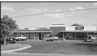
8007 Mechanicsville Tpk 9,669 SF Lease - $10.50 MGRS Bill Mattox
