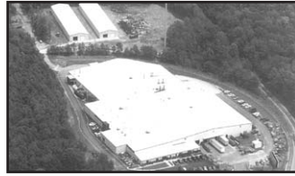
Waverly Textiles 8401 Fort Darling Road 136,017 SF Sale $3,157,925 - Lease $3.25 Bill Mattox, Jason Hetherington
