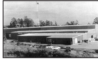
14500 Jefferson Davis Hwy 36,000 SF manufacturing with crane Sale - $1,380,000 Lease - $11,850/mo NNN David Williams
