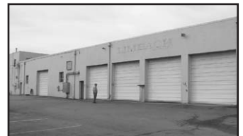
Mechanicsville 2415 Anniston Street 9,186 SF Lease - $5.50 NN Jason Hetherington
