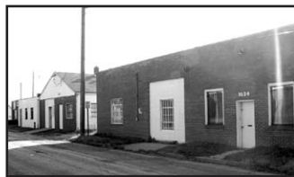
NEW 1532-34 High Street 14,006 SF Built out as office Lease - $5 - $7 MGRS Jim Ashby, Garnett Hall
