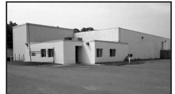
9975 Lickinghole Road 13,900 SF Includes 20x40 Subzero Freezer Lease: $5.25 - 7.10 NNN Stuart Cary, Jason Hetherington
