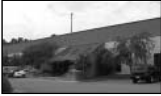
Telecommunications Center 10436 Wilden Drive 64,064 SF Sale - $3,300,000 Dawn Carson, Stuart Cary, Steve Gentl
