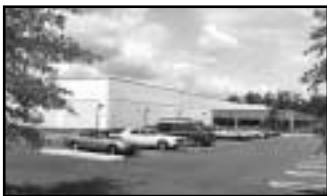
Villa Park Tech Service Center 8000 Villa Park Drive 108,000 SF Sale - $6,600,000 David Williams, Bill Mattox Steve Gentl
