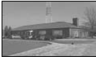
Flex Building - Dabney Area 2100 Maywill Street 6,790 SF Lease - $7.75 NNN Jason Hetherington
