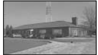
Flex Building - Dabney Area 2100 Maywill Street 6,790 SF Lease - $7.75 NNN NEW Jason Hetherington
