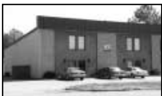
Office/Production/Warehouse 205 Haley Rd, Ashland 11,100 SF Lease - $5.50 NNN Dawn Carson, Stuart Cary
