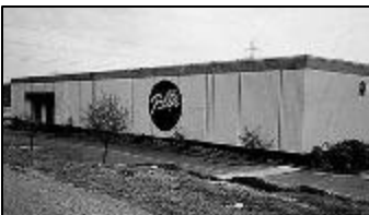
2211 Station Road (Chesterfield) 11,850 SF Lease - $3.75/SF NNN Jason Hetherington
